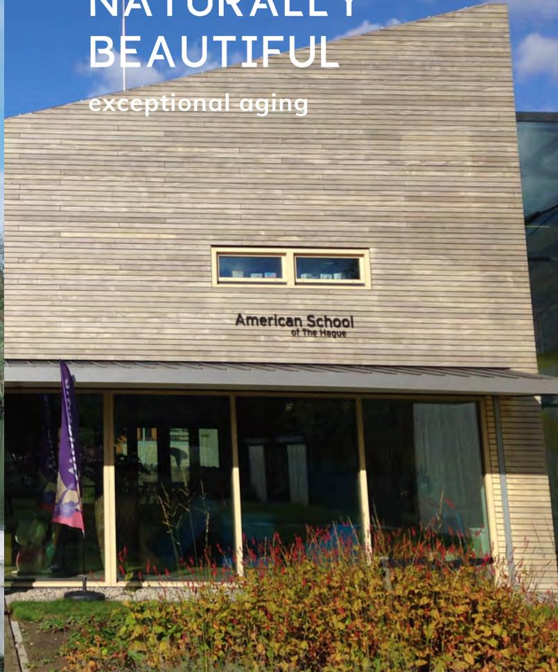
The durability (resistance to rot) of Accoya wood is Class 1, exceeding commonly used cladding woods such as Western Red Cedar, Larch, Douglas, tropical hardwoods and thermally modified woods. Each batch of Accoya wood is analyzed in the laboratory after production to guarantee its performance.
